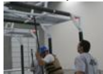
Ceiling Breach & Pull
